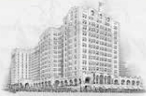
BOARDWALK AT BRISHTON AVE.
